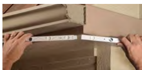
Fit Magnet Tracks together, change magnet spacing on back.
