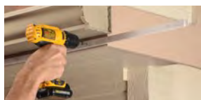
Attach with screws (permanent) or 3M Double stick tape (temporary) included.
